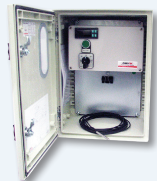
Milk Vat Control Panel with viewing window as standard
